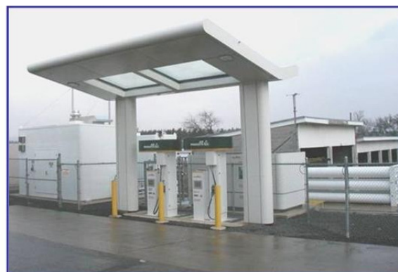
Figure 3.1.1 Distributed hydrogen production facility
